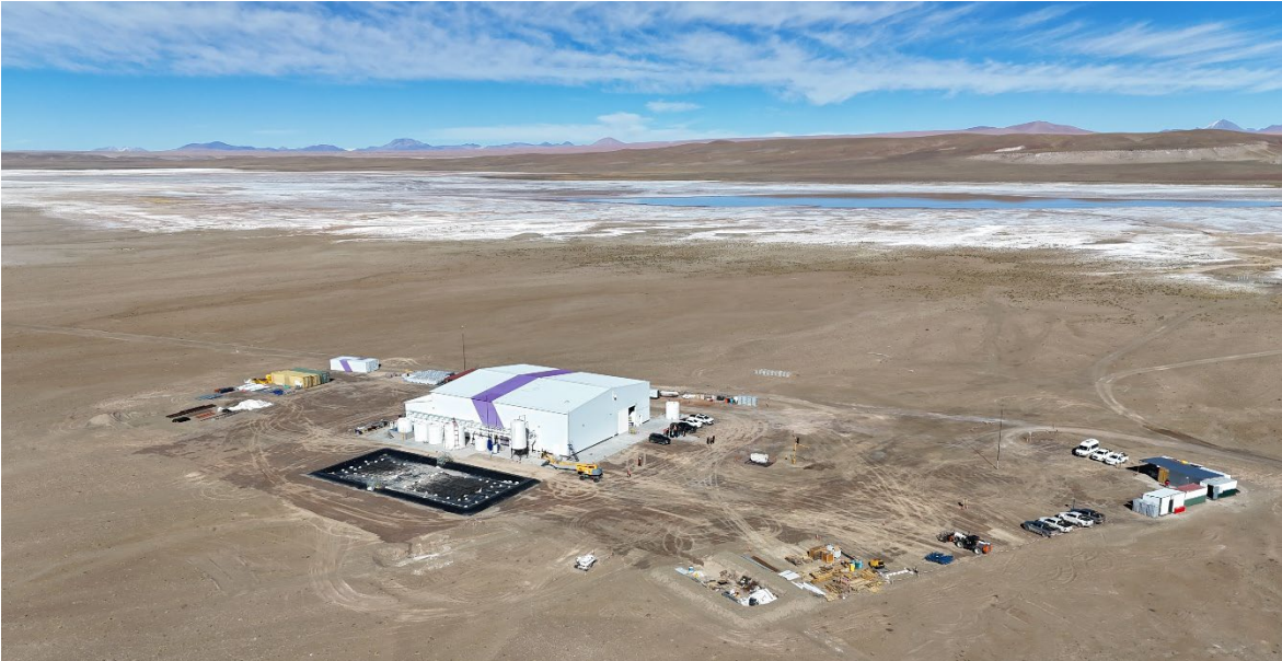
DEMONSTRATION PLANT, JUJUY PROVINCE, ARGENTINA, EXTERIOR
