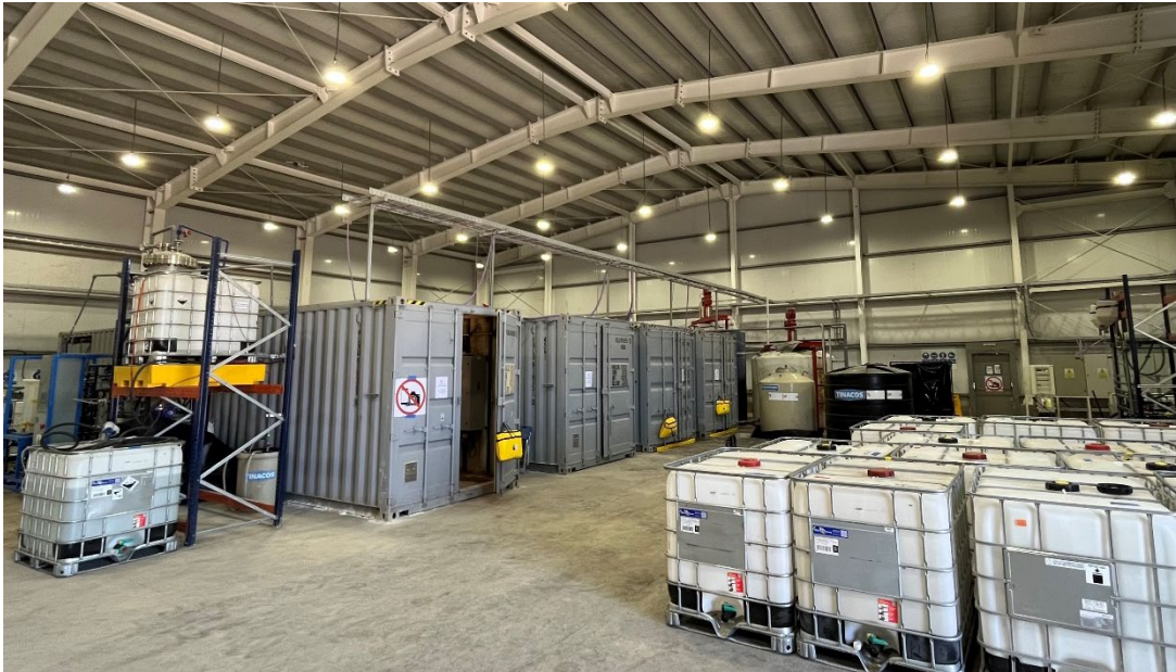
KACHI DEMONSTRATION PLANT, CATAMARCA, ARGENTINA, INTERIOR
