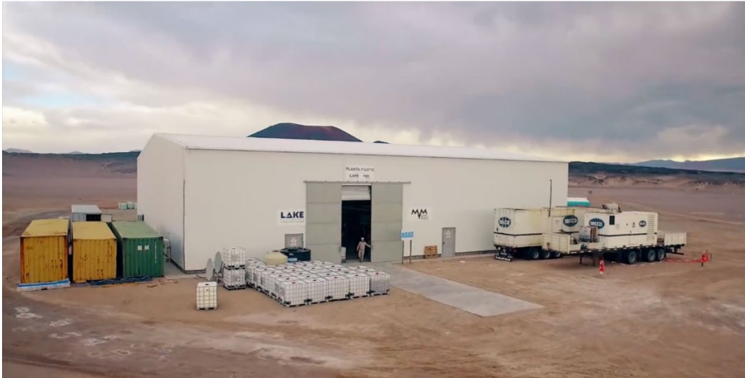
KACHI DEMONSTRATION PLANT, CATAMARCA, ARGENTINA, EXTERIOR
